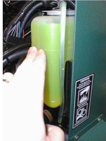
2. **Weekly**, remove the radiator cap and check the coolant for proper level. This level should be approximately 1/2 inch from the top.
